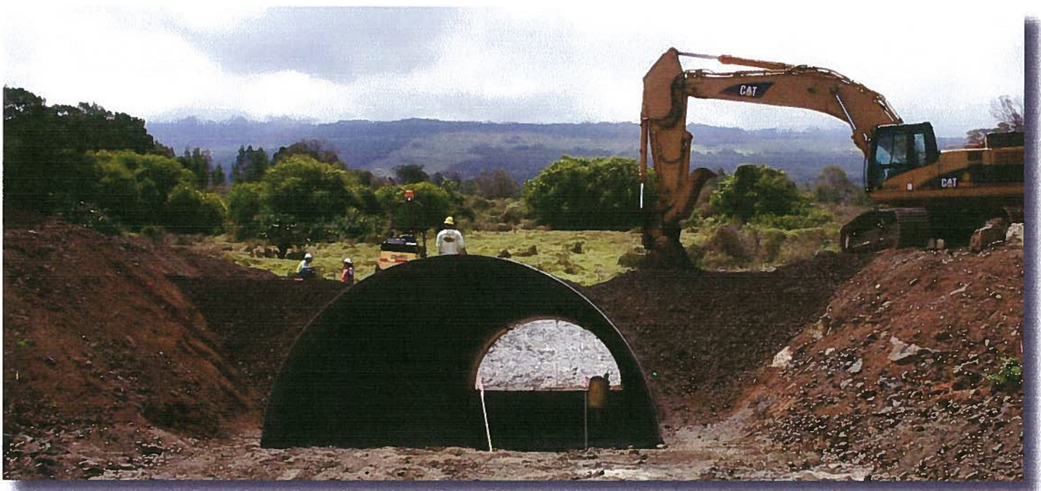
Infrastructure work at Waiohuli, Maui.
