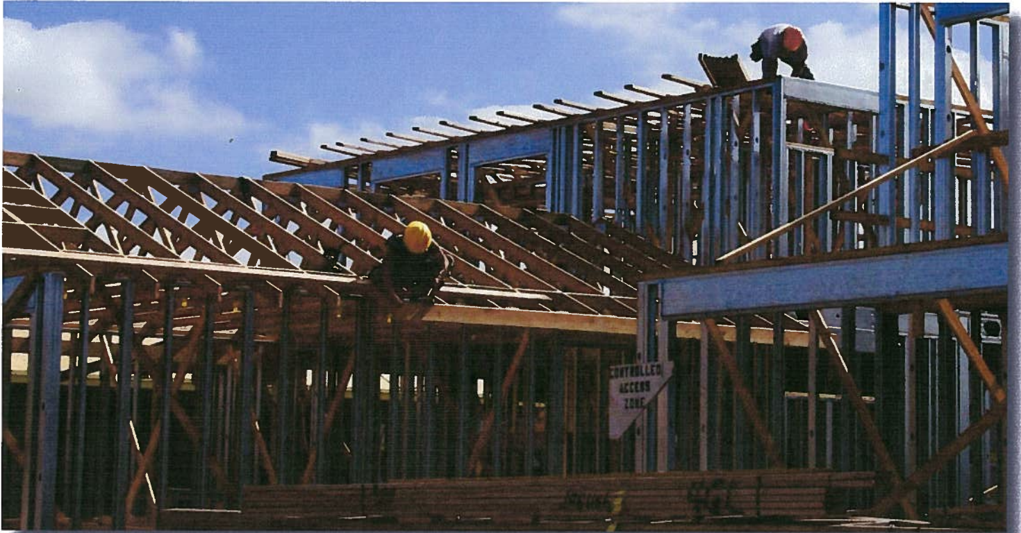
Home construction at Kaupē'a, O'ahu.
