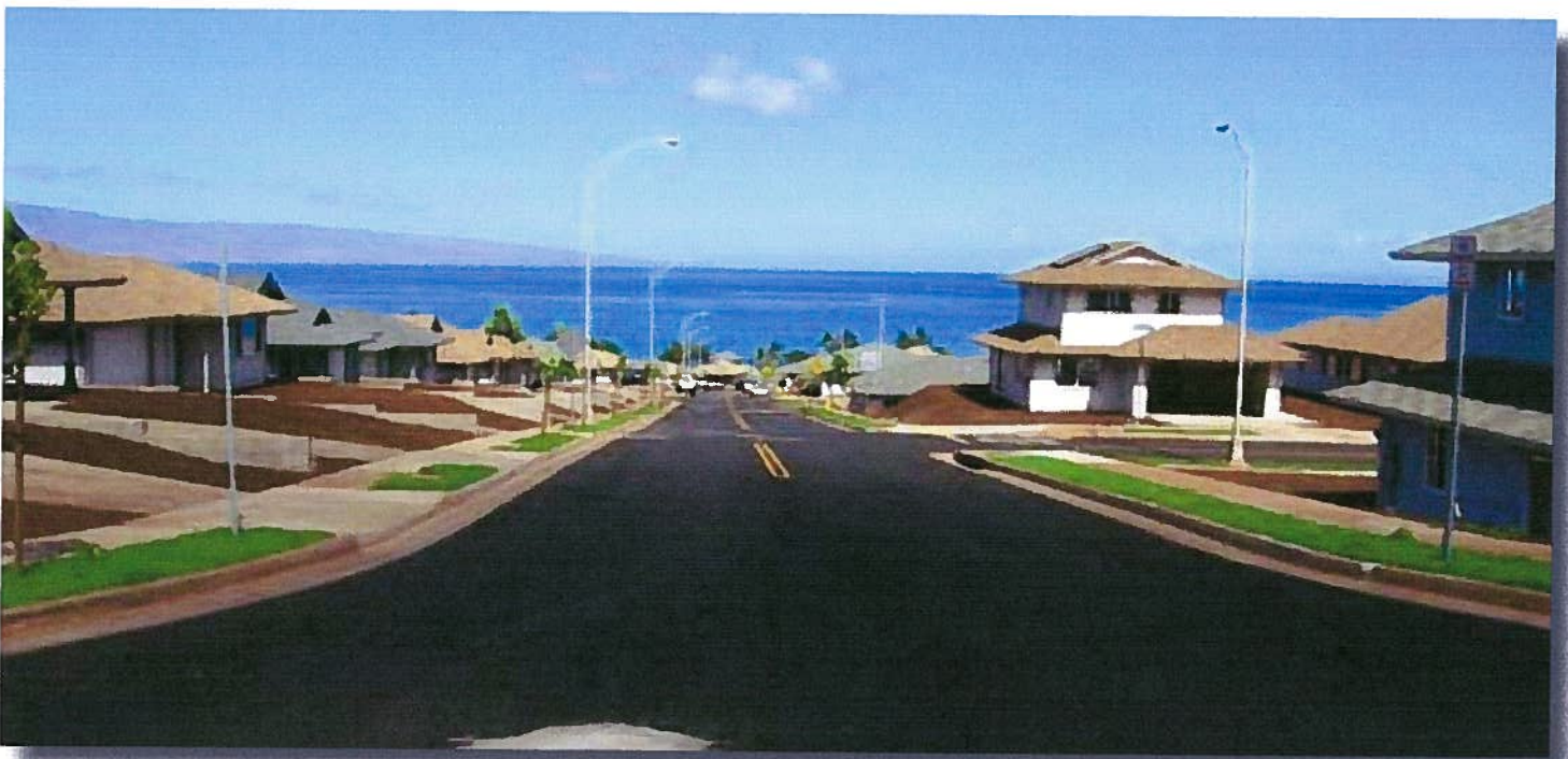
Completed homes at Leiali'i, Maui.
