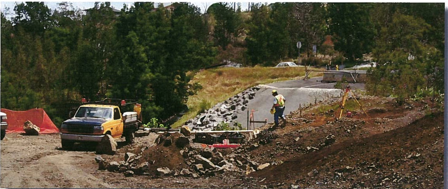
Roadwork at Waiohuli, Maui
